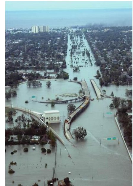
Hurricane Katrina, New Orleans, 2005
